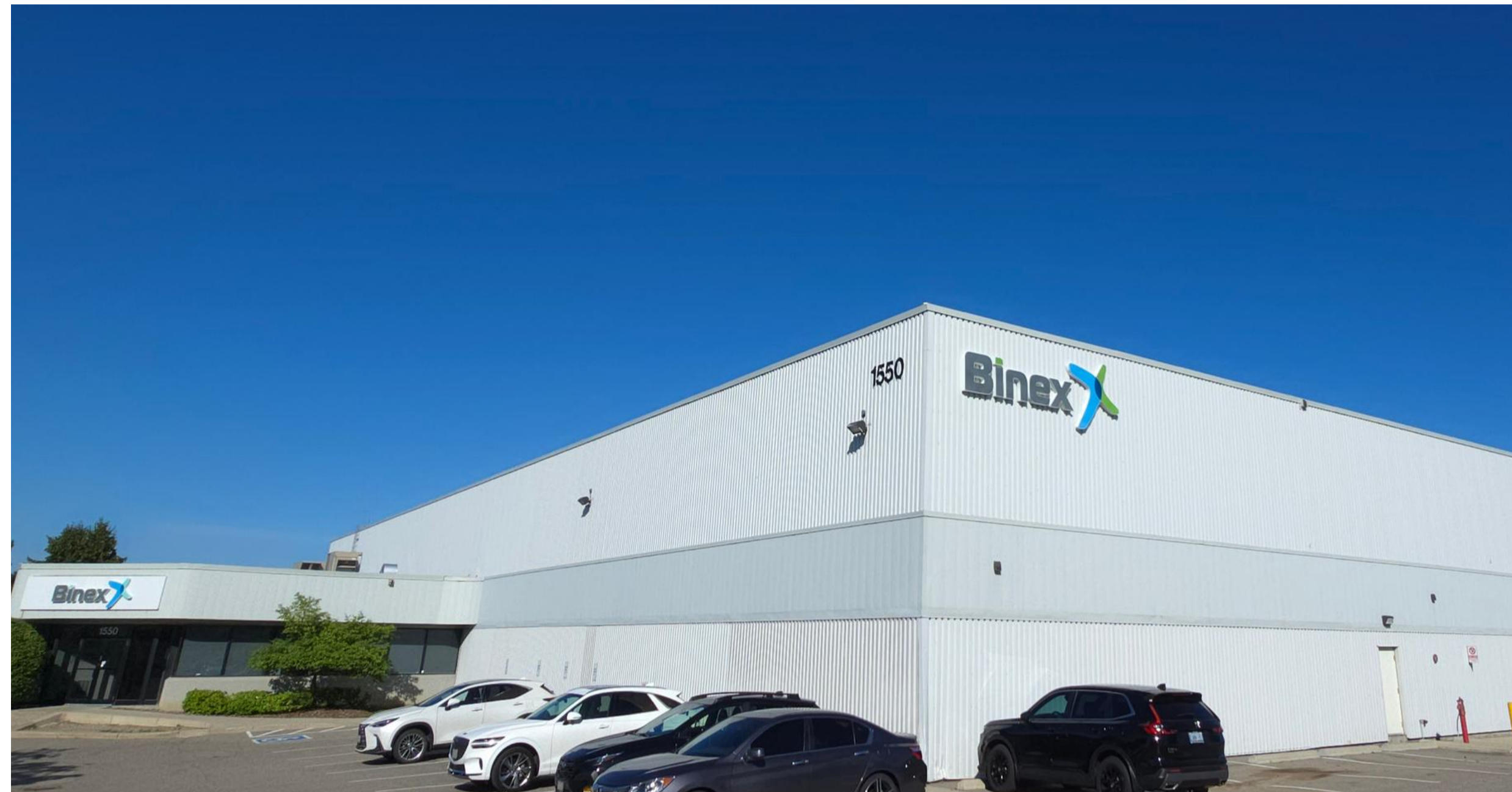
Toronto Warehouse & Office
