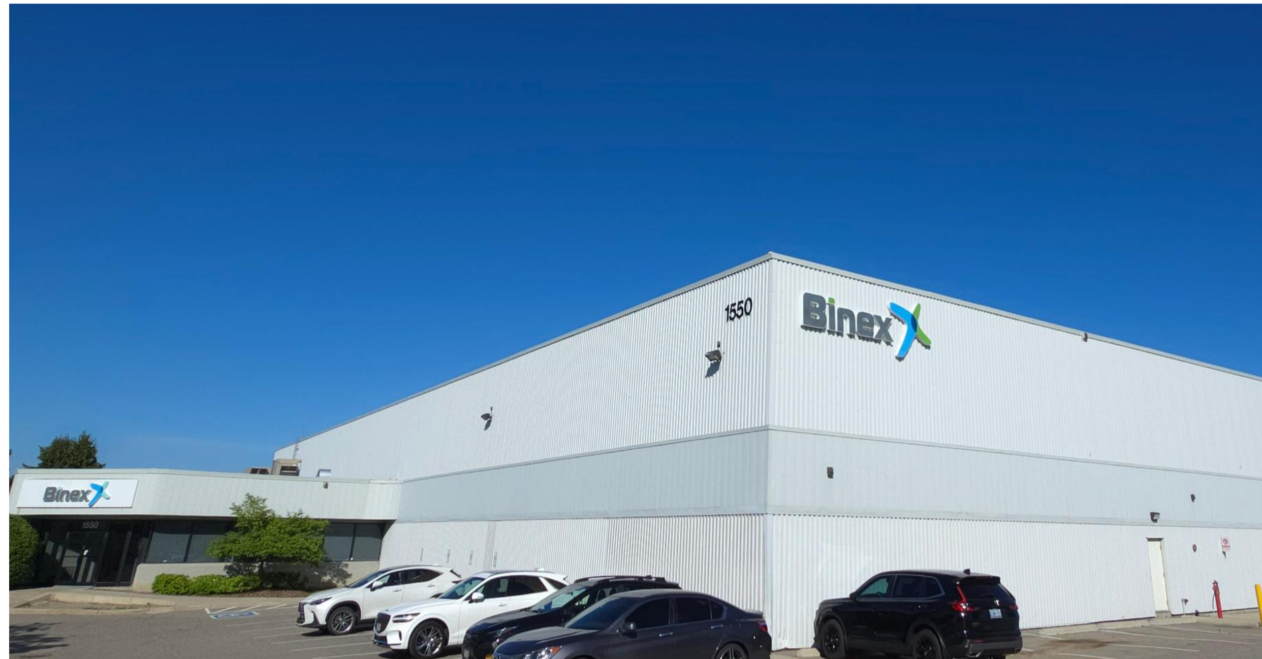
Toronto Warehouse & Office
